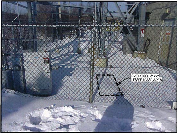
PROPOSED EQUIPMENT LOCATION - LOOKING NORTHEAST -
