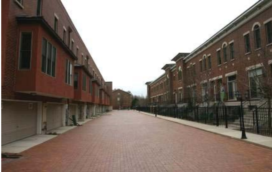
Image 8 shows residential units facing garages. This should not be allowed in the corridor.
