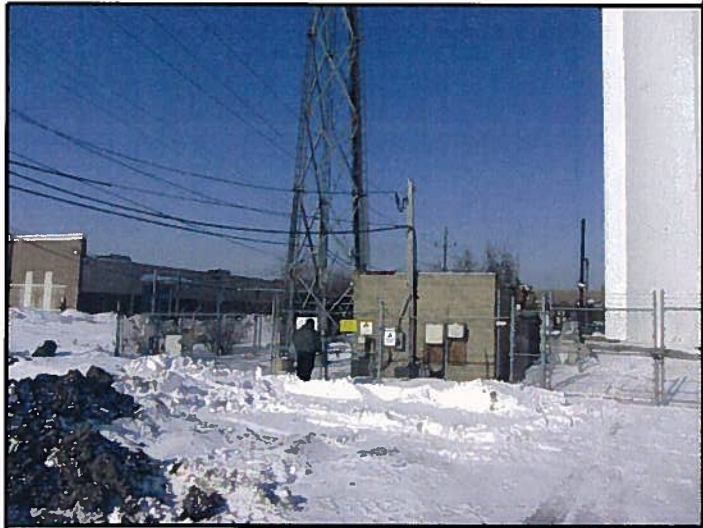
SITE OVERVIEW - LOOKING NORTH -
