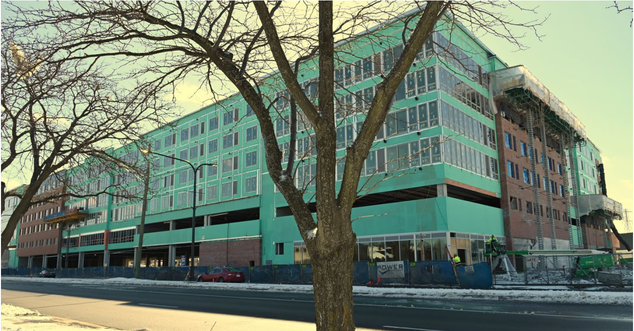
District 1860, redevelopment of approximately 9 acres at the corner of Touhy Avenue and Lincoln Avenue.
