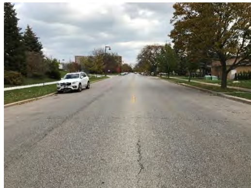
Average Pavement – Resurfaced in 2011 W. Pratt Ave (E. of N. Crawford Ave)
