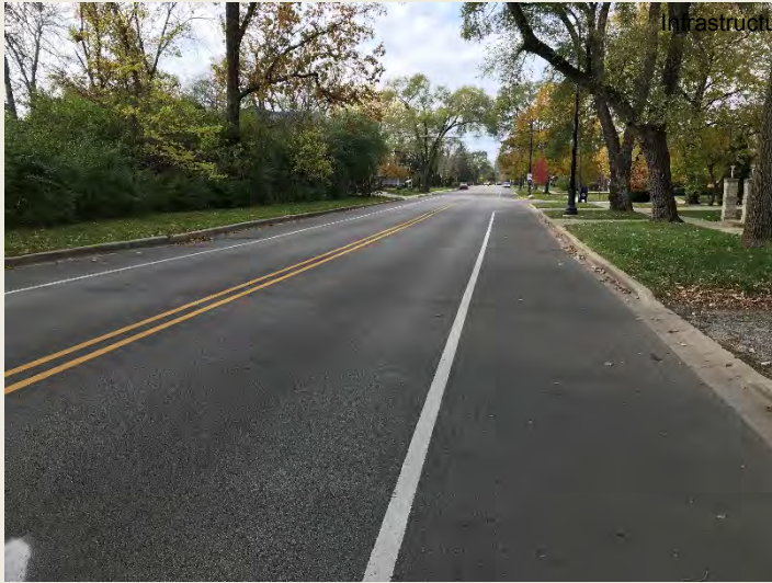
Good Pavement – Resurfaced in 2016 W. Pratt Ave. (W of N. Crawford Ave.)
