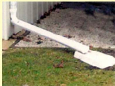
Correct: Disconnected Downspout (picture above)
