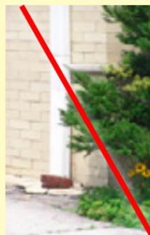
Incorrect: Connected Downspout, in violation with Village Code (picture on the right)
